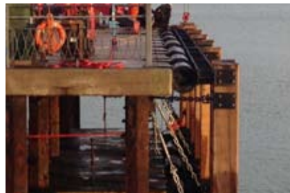
Repairs finished at Llandudno
